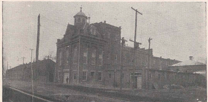
Virginia Brewing Co.'s Plant
