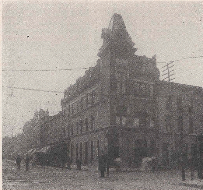
Campbell Avenue, Looking West
