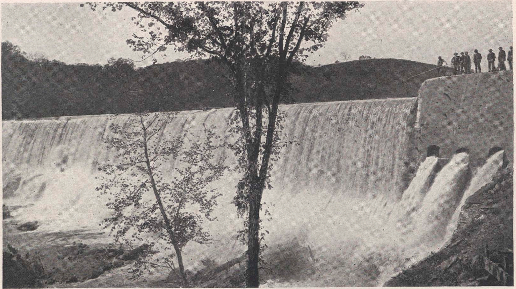
Dam of the Roanoke Water Power Company
