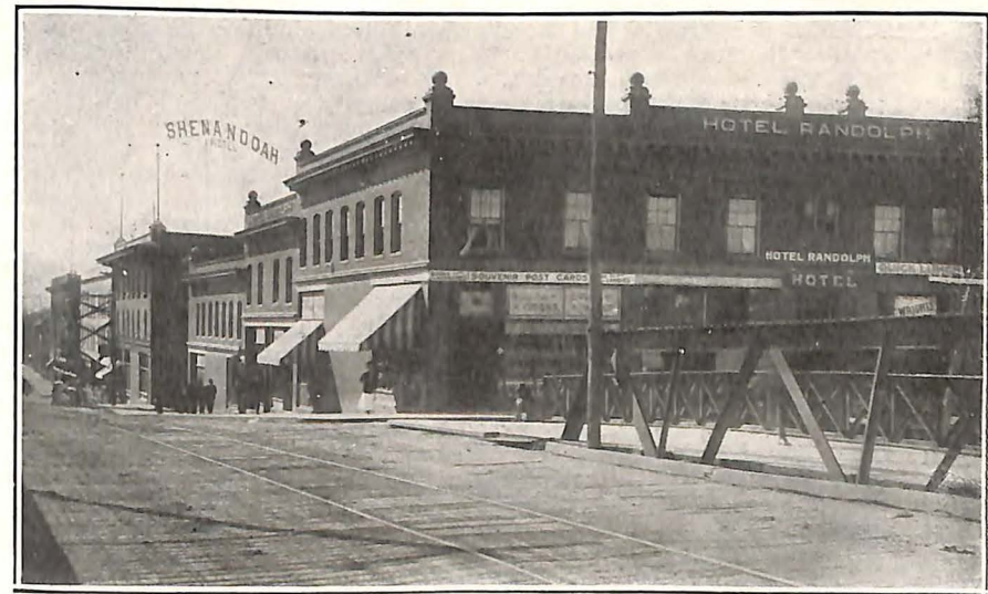
Randolph Street—Viaduct Crossing at Norfolk & Western Passenger Station
