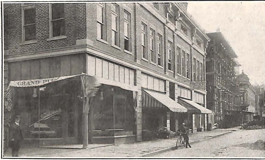
Henry Street, Showing New Post Office in Course of Construction Grand Piano Company in Foreground
