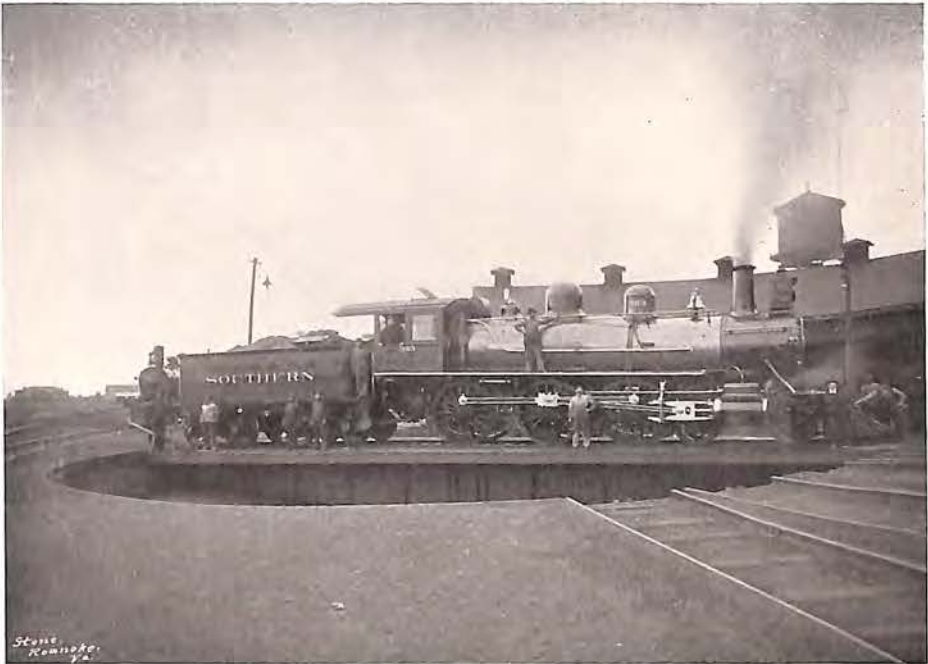
SIXTY-FIVE FOOT DECK TURNTABLE FOR 300,000-POUND LOCOMOTIVES. BUILT FOR SOUTHERN RAILWAY COMPANY, AT SALISBURY, N. C.
