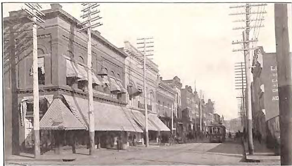
CAMPBELL AVENUE, LOOKING EAST FROM S. H. HEIRONIMUS & CO.'S STORE
