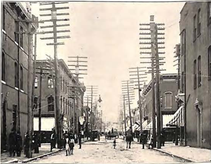
Salem Avenue.—Looking West.
