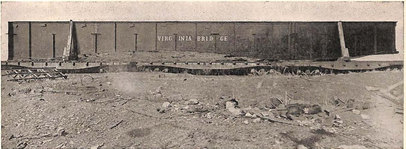
This steel girder, 120 feet in length, and requiring three flat cars for transportation, was manufactured by the Virginia Bridge and Iron Company for the Spring Street viaduct, Atlanta, Georgia.
