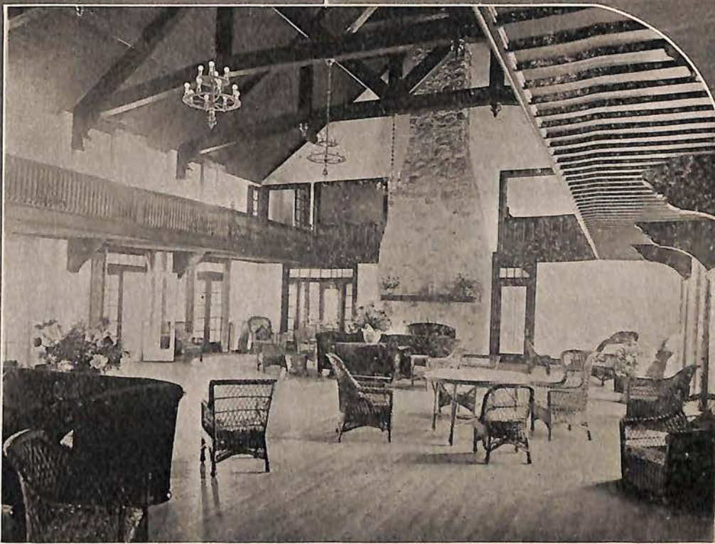
Interior view of Clubhouse
