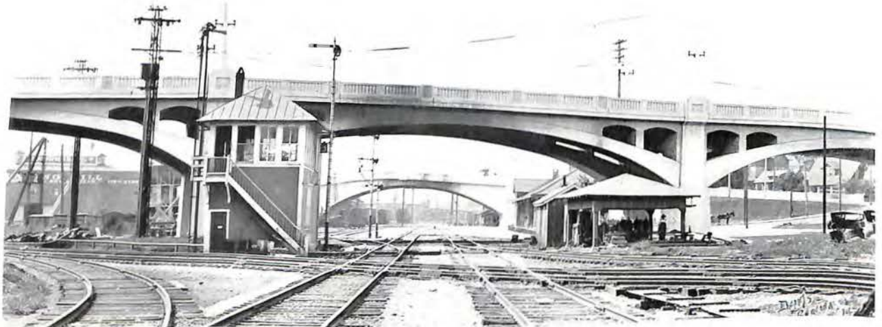
SIDE VIEW OF THE NEW WALNUT AVENUE AND JEFFERSON STREET BRIDGES OVER THE NORFOLK AND WESTERN AND VIRGINIAN RAILWAYS
