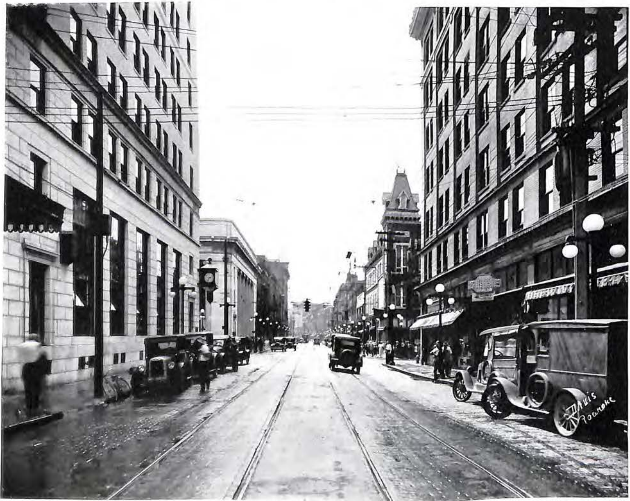
CAMPBELL AVENUE, LOOKING WEST In the business section of the city
