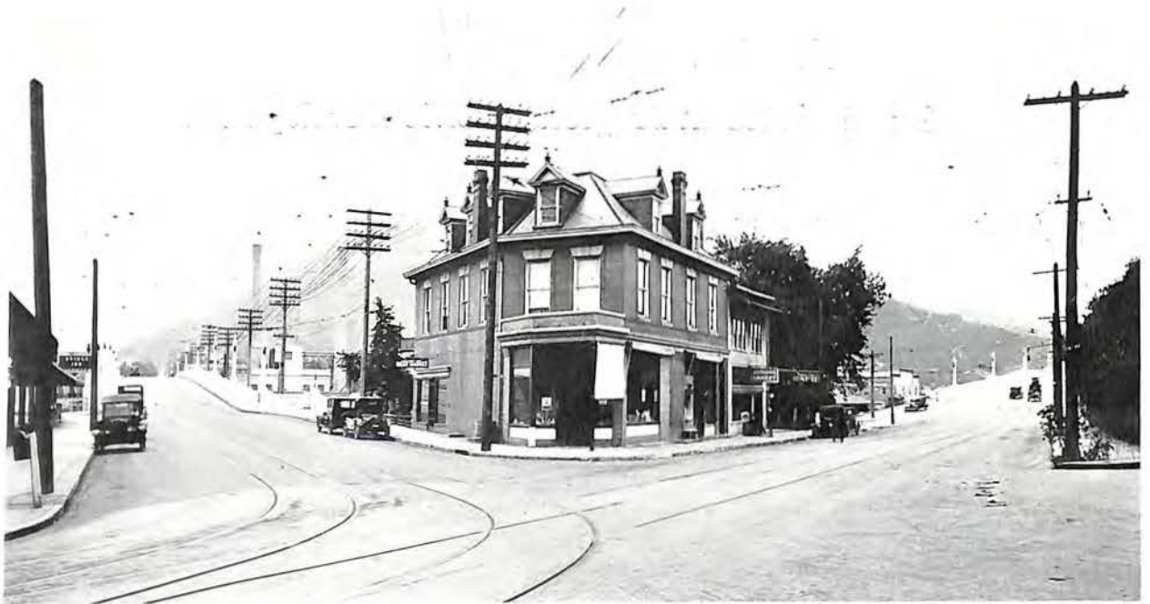
APPROACHES TO THE TWO NEW BRIDGES ON WALNUT AVENUE, LEFT, AND JEFFERSON STREET, RIGHT, OVER THE NORFOLK AND WESTERN AND VIRGINIAN RAILWAYS
