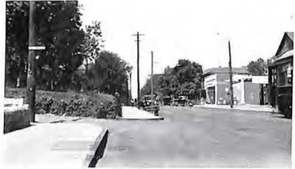
CAMPBELL AVENUE IS GRADUALLY BEING WIDENED
