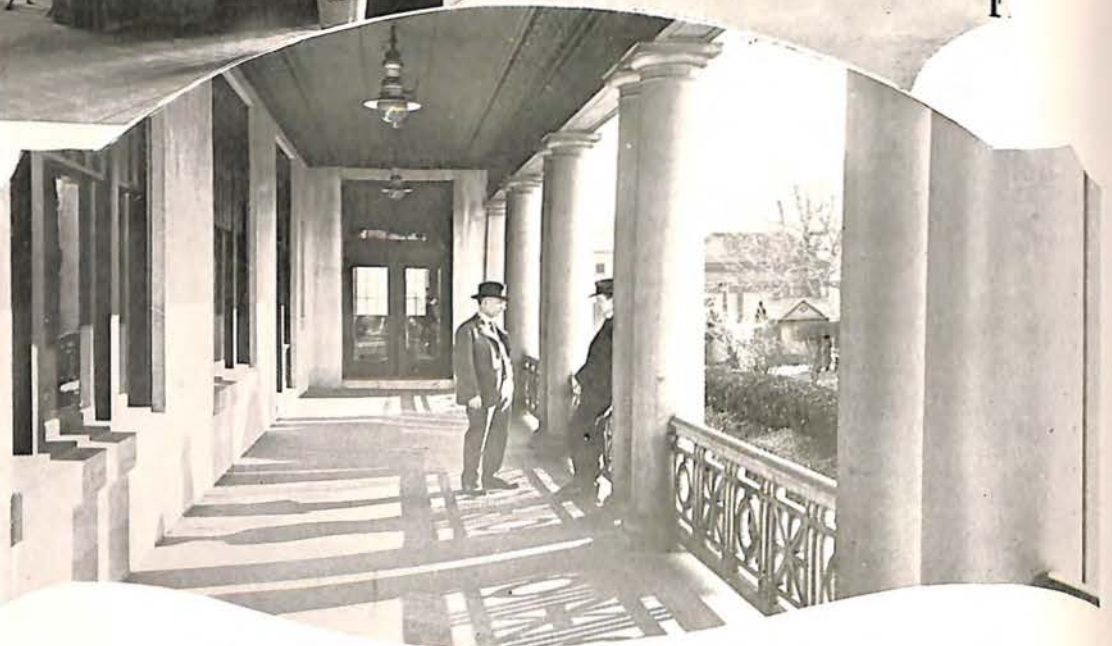
Entrance and Partial View of Auditorium
