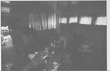
David Shepard Sr.'s house at 1824 Melrose Ave. N.W. was trashed by a tenant last summer. He found a charcoal grill in the middle of the living room, mattresses left in the bedrooms, food rotting on the kitchen table and a broken window on the front porch. Shepard said the tenant moved out without a word, owing him rent.
