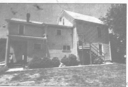
This house on Loudon Avenue northwest (above) was one of the first to be fixed up by the Northwest Neighborhood Environmental Organization. The same house before renovation is seen below.
