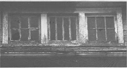
Neighbors said this house on 14th Street Southwest has been vacant since shortly after its last occupant was taken into custody several years ago.
