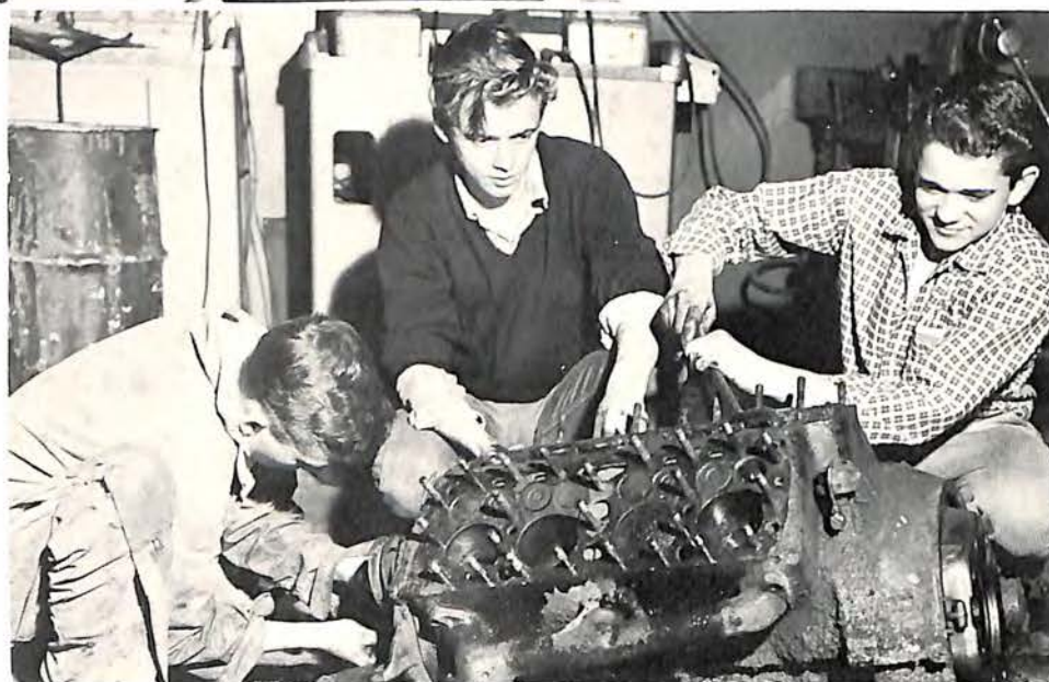
Eugene Davis, David Martin, and Donny Poff tear down an engine as part of the Auto Mechanics training class.
