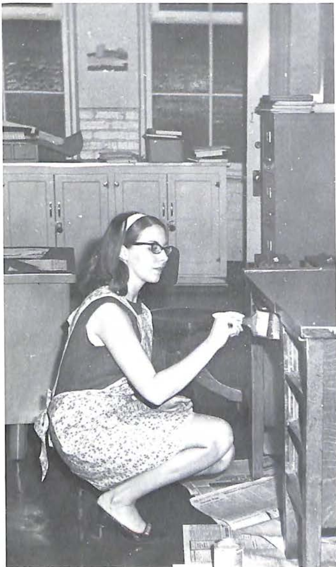
Mrs. Rita Wilson appears to be into the task of beautifying the office with a new paint job.
