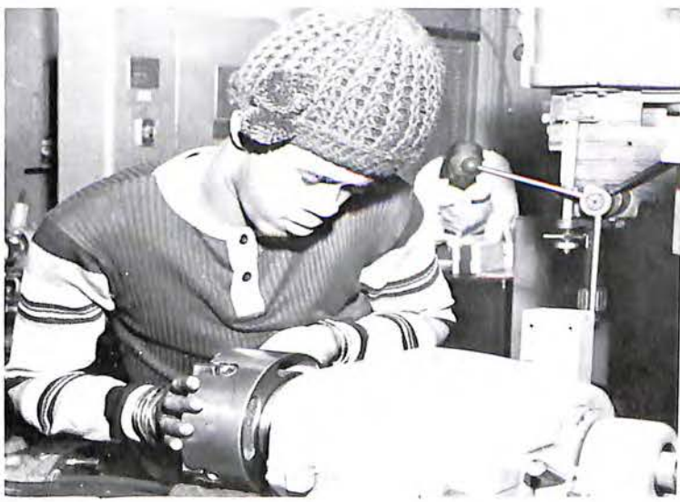
Jimmy Saunders is putting a chuck on an engine lathe.
