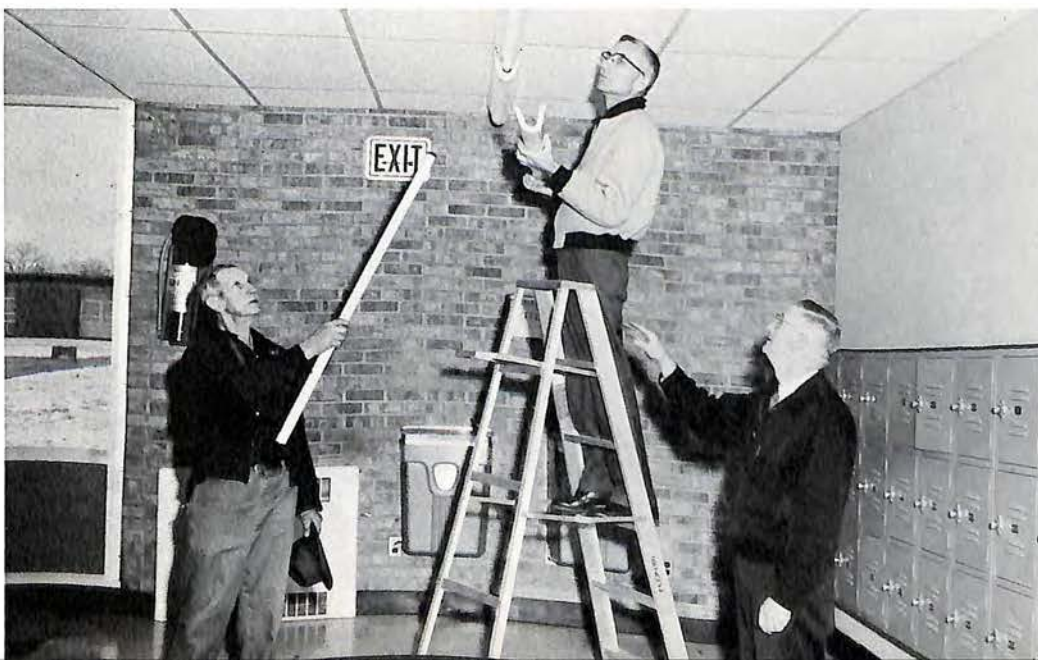
Fleming's custodial staff, Mr. Paitsel, Mr. Woodford, and Mr. Lugar, repair light in Smith Hall.
