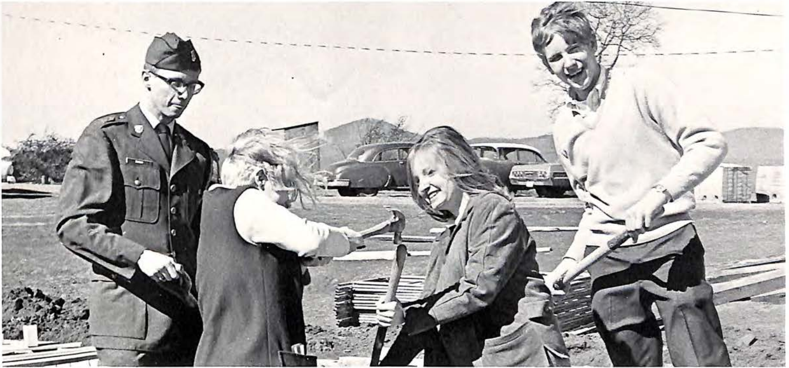
WE SHOULD HAVE THIS HALL UP IN NO TIME . . . Students help build the new hall in free afternoon hours.
