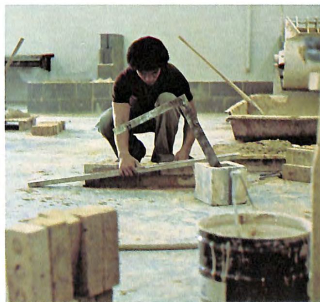
Leveling off. Junior Charles Thomas checks the lay of his bricks during masonry class.
