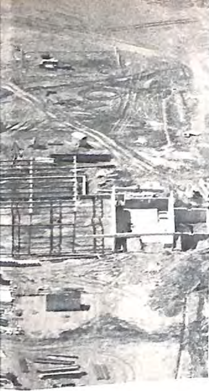
An airview look shows Patrick Henry High School under construction last summer.
