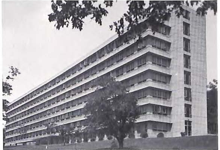
Hospital Catawba Sanatorium
