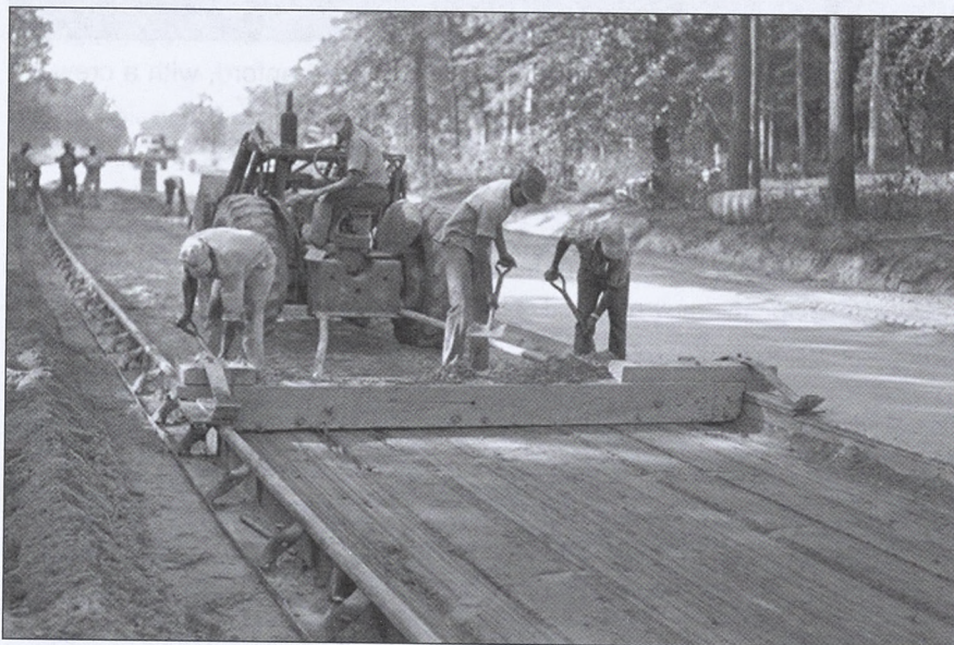
Workers prepare forms and subgrade for concrete pavement.
