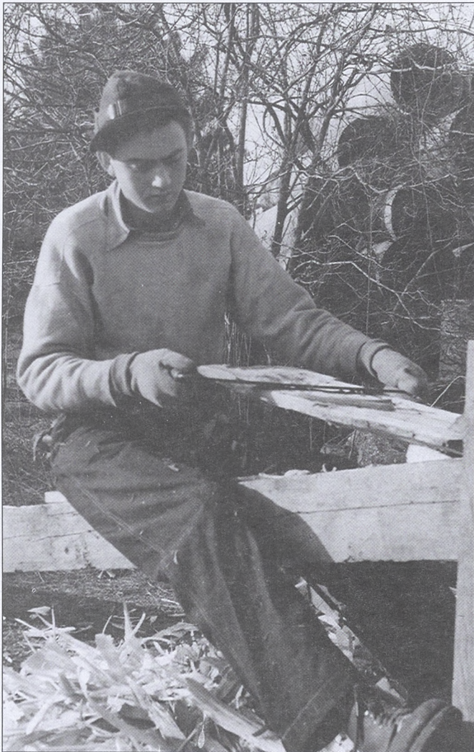
A worker uses a drawknife to smooth and taper a plank.
