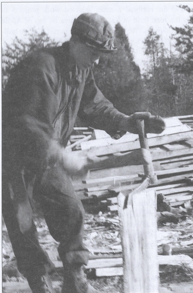
With a wooden mallet and a froe, a CCC worker splits a block of wood.
