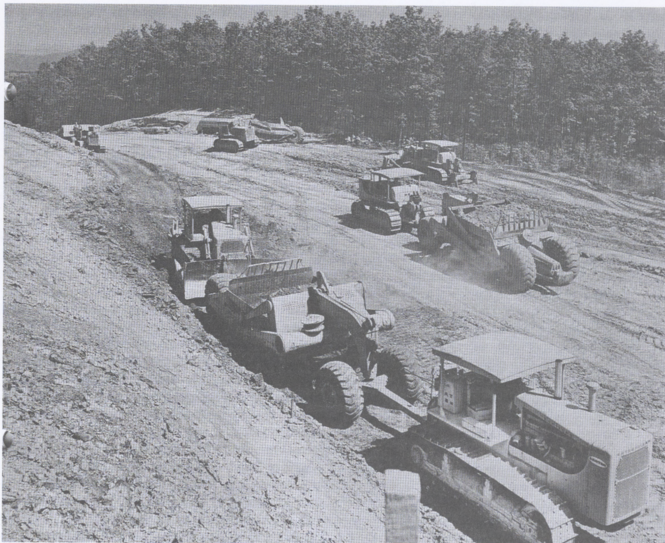
Robertson, Fowler and Co.'s big scrapers are working on U.S. 460 at the top of Brush Mountain north-west of Blacksburg. (Virginia Road Builder magazine, Volume XXIII, No. 11, June 12, 1967)
