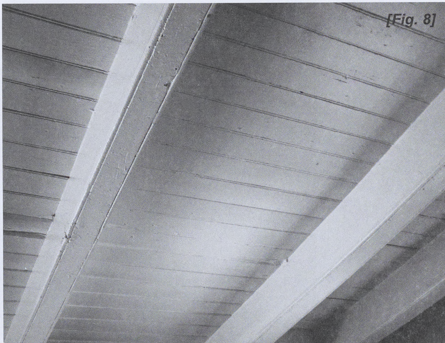
Fig. 8. Hand-planed, beaded floor boards, nailed to hand-planed, beaded joists, which suggest a pre-1840 construction date.
