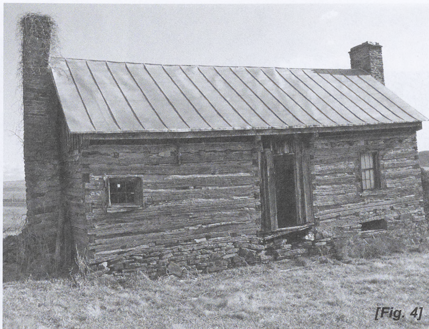
Fig. 4. Ivy Cliff servant quarters (ca. 1840-50) in Bedford County, provide a good example of a one-story, dogtrot house with square-notched logs.
