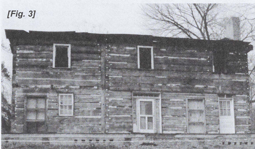
Fig. 3. The Howbert House, a substantial, two-story structure demolished in 1999, stood near the intersection of Salem Turnpike and Peters Creek Road in Roanoke. The smaller, V-notched pen (left) was added to the larger, full-dovetail-notched pen using two 8"x 8" corner posts abutted to the original structure. The front- and rear-wall logs of the added pen were then mortised into the corner posts. (Photo credit: Anne Beckett)
