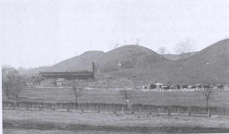
Figure 8. The Scott Furnace seen in 1893. Furnaces were long, shed-like buildings with a large chimney at one end. This facility fired 440 kettles in two double furnaces and supplied the Confederate States Army with salt. (Phillips-Perry Collection, picture a42, courtesy the Museum of the Middle Appalachians)
