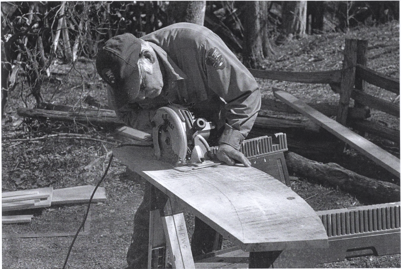
Jack Trivett cuts a white oak board to make a replacement part for Mabry Mill's century-old water wheel. All the restoration work was done on-site.
