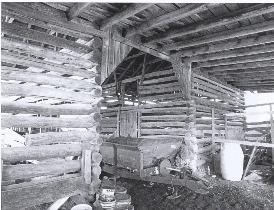
The double-crib log barn on the Key-Shackford Farm probably dates to the 1910s or 1920s but is representative of earlier log barns.
