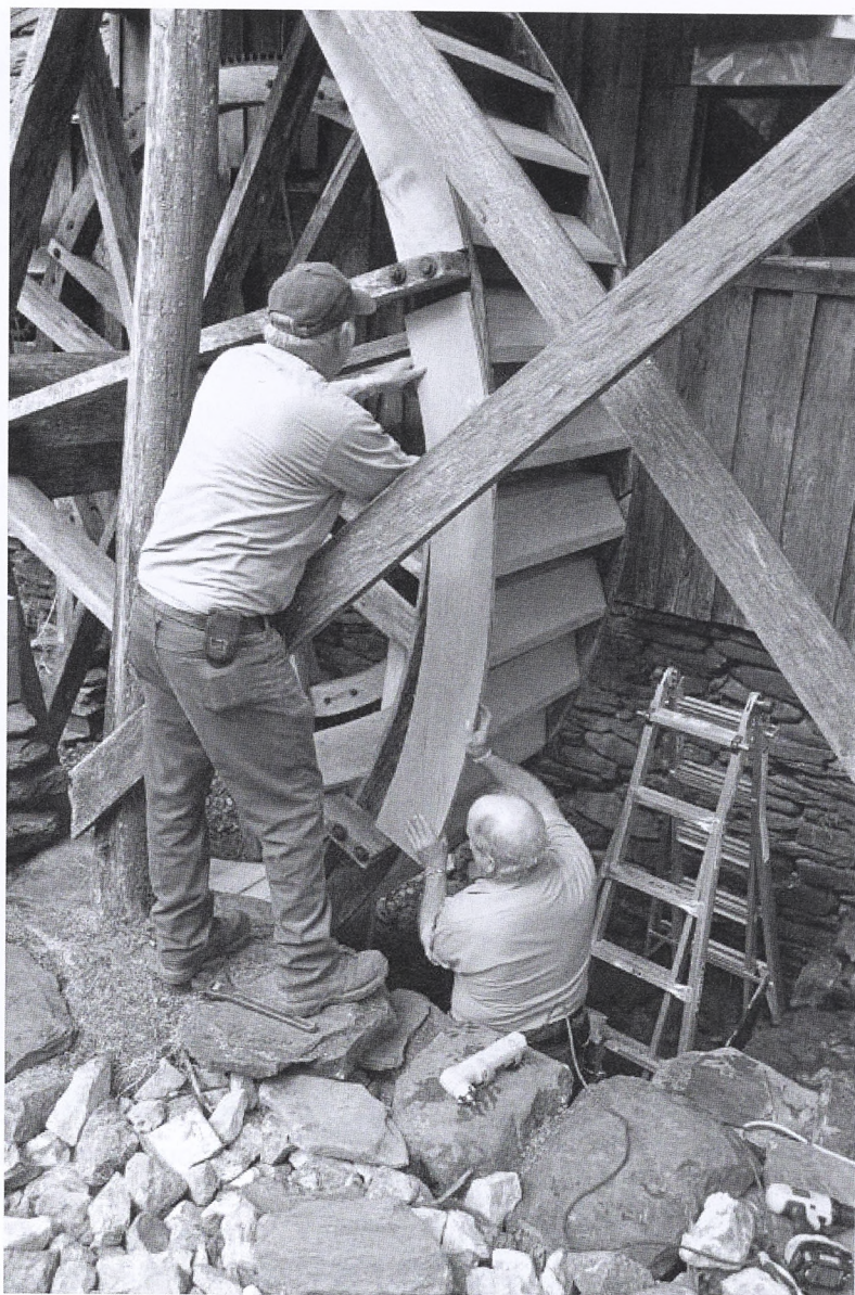
Jack Trivett (left) and Steve Marmie fit one of the newly fabricated parts onto the waterwheel. The replacement wood came from a fallen tree estimated to be 400 to 500 years old.
