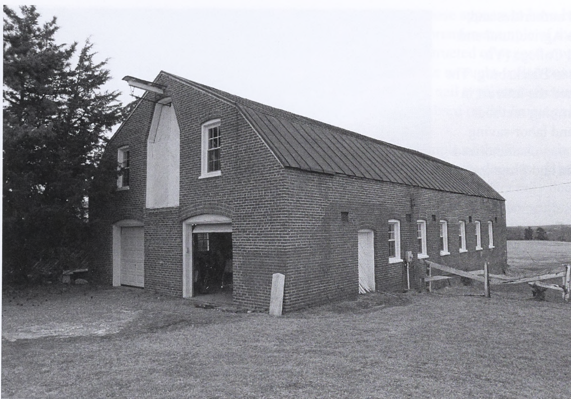
The brick horse barn at Savenac is an early local example of the gambrel-roofed form.
