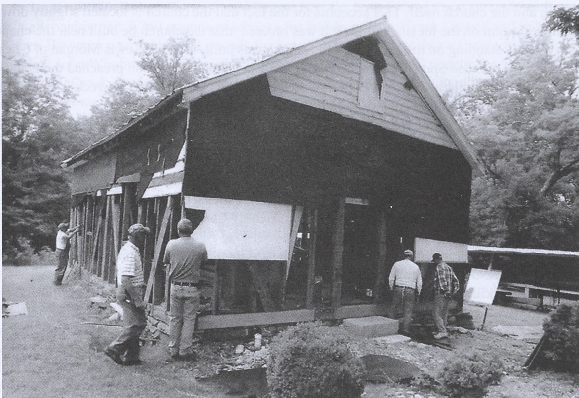
Restoration scene at Old Chapel Church. Notes with this photograph say, "Reproduction 18th century nails used for cypress beaded weatherboards." (All photos by Dr. J. Francis Amos)
