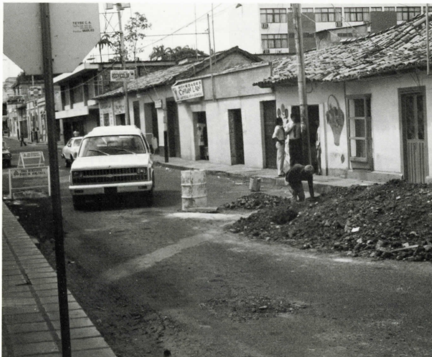
Work is done on a sewer connection for a new building in San Antonio, Tachira, with a surprising lack of barricades.
