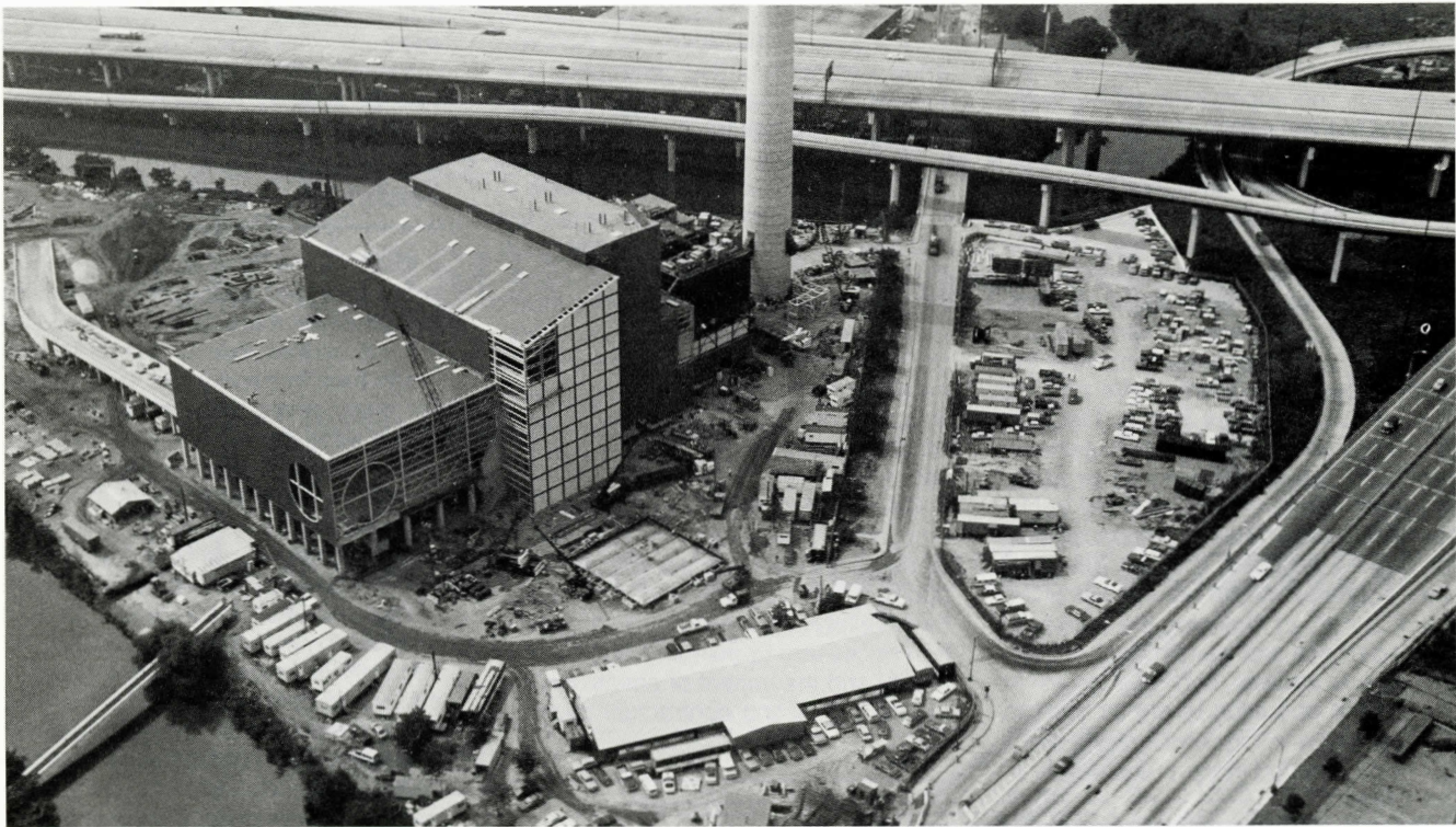
The Southwest Resource Recovery Facility, a recently completed privatization project constructed in Baltimore, burns 2,000 tons of garbage a day converting the waste into steam, electricity and other usable material.
