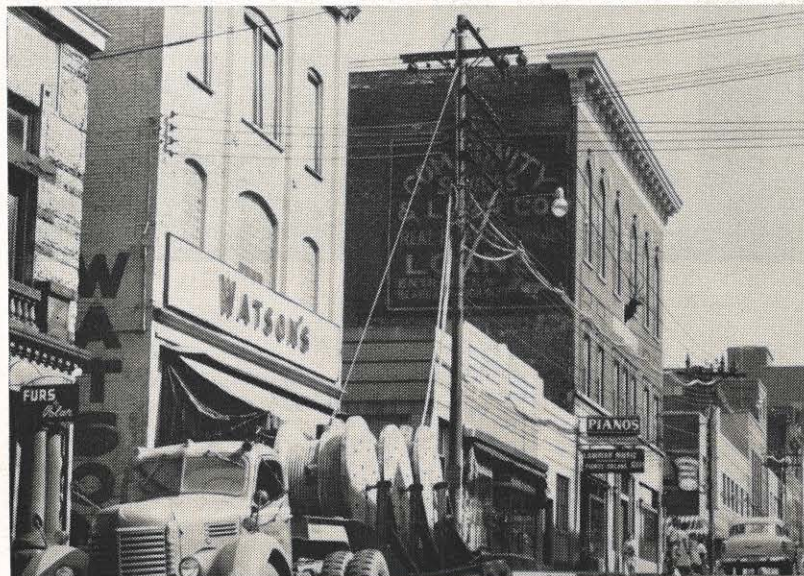
Aerial cable is being installed in Bluefield's downtown section. Here the cable has been carried to the pole in back of the truck. Most of the crossarms on that pole and others will be removed later.
