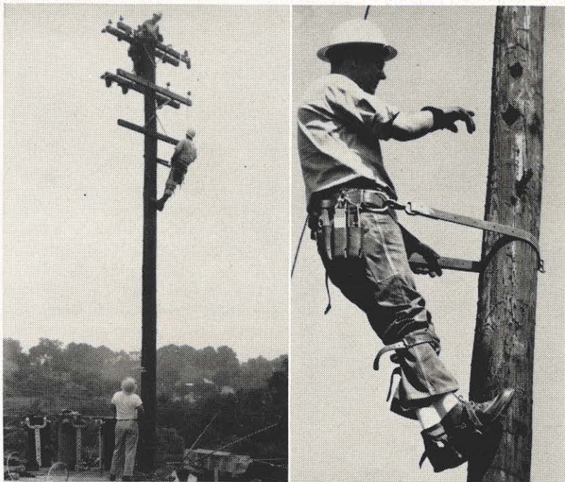
LEFT: This pole is being prepared to receive three 37½ Kva transformers to serve a new commercial customer in the Lynchburg district. Work on poles is carried on constantly in our three companies. Shown are from top to bottom: Sandidge L. Drumheller, lineman; James E. Howard, lineman; and James A. Martin, groundman. RIGHT: Willie E. Metts, general serviceman, points to woodpecker holes 15 feet up on a wood pole. Woodpeckers are second only to natural rot and decay in destroying utility poles. Most of the damage by woodpeckers is done higher up on a pole than these holes, usually in the vicinity of the crossarms.
