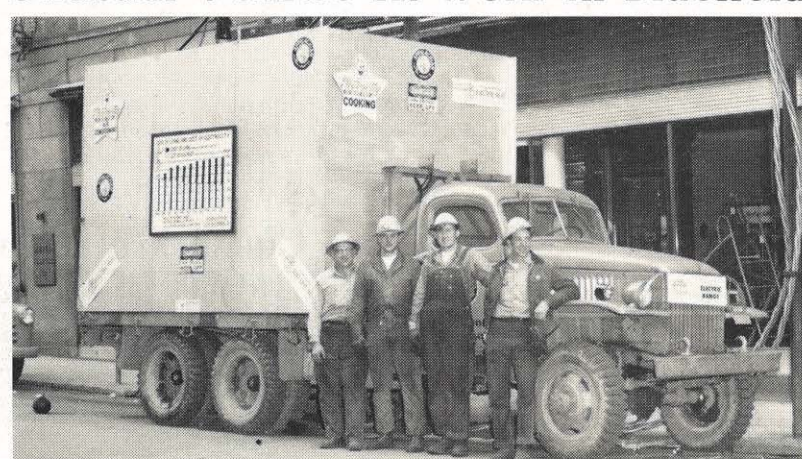
Bluefield substation crew members line up in front of an unusual vehicle called the "vault-wagon." From the left are R. H. Stowers, Jack Spraker, Ray Eskew and R. R. Jones. The vault-wagon contains three 100 kva transformers that take the place of underground equipment being changed from 4 to 12 kva. It is driven to a point near the vault and replaces it for two or three days while the work is being completed. The wagon, built by Bluefield substation men, is encased in plywood as a safety measure and features company promotional material on its sides.
