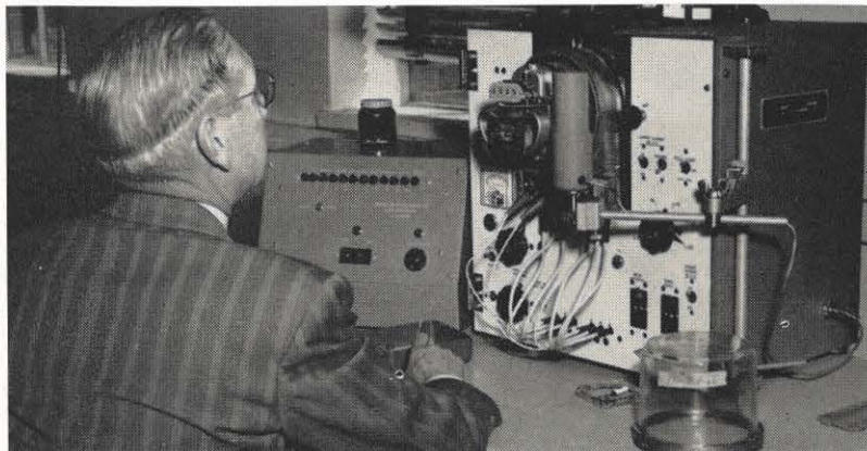
Using another precision instrument in the Roanoke meter department, C. A. Farrar, meterman, tests a three-phase watt-hour meter.
