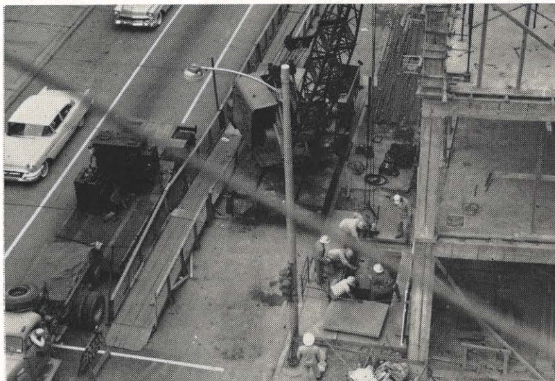
Expansion of the Charleston underground system in 1957 was virtually complete when two transformers were installed last month. Crews headed by Mike Shafer and Steve Didier are shown installing a transformer in the vault alongside the J. C. Penney store, under construction. This picture, taken from the seventh floor of the Daniel Boone Hotel, also shows another transformer on the truck. This one was also installed.
