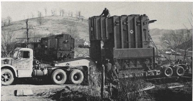
Preparing to make a mile-long trip from a railroad siding at North Tazewell to its destination at the Tazewell station is this 58-ton transformer. The 40,000 kva three-phase transformer, which will step power down from 138,000 volts to 33,000 volts, will provide for present and future growth at the Bluefield district station, as well as give additional voltage regulation in the area. The transformer, which weighs 58 tons without oil or bushings installed, was transferred from the railroad car to the truck, and then set on its base at the station with the help of a giant bulldozer. J. G. Tapley, system senior station engineer, is the company engineer in charge of the station work.
