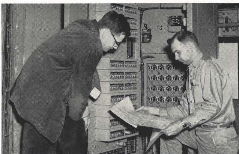
Through this relay system, electrical instructions are fed to Buck hydro plant generators from the Byllesby plant, two miles away. Checking the equipment are Foster Janich, left, from the company that supplied the equipment and Leroy Dalton, Pulaski district meterman.
