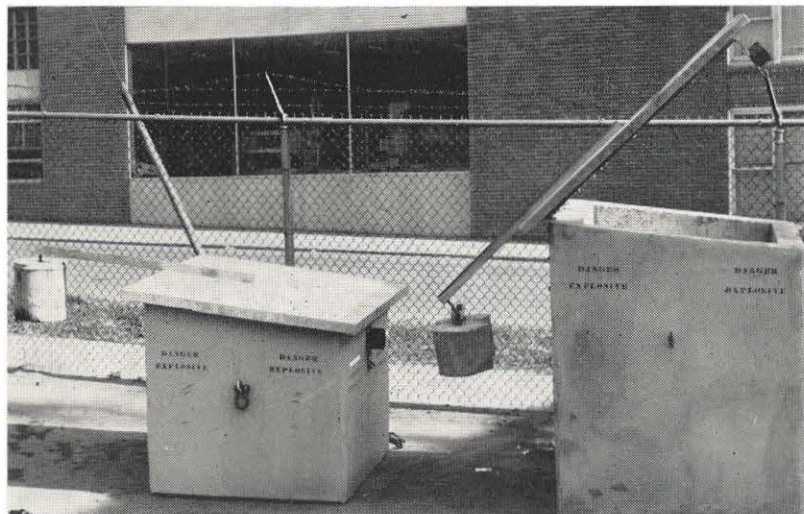
The newly designed and built dynamite magazines in the Bluefield district come in two sizes. They are portable, safe and convenient. Shown here are the counter-weighted lid and enclosed hasp, both safety features.
