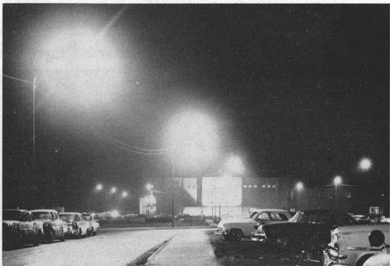
The new high school and fieldhouse at Logan are wearing a new night-time look. Modern street lighting was installed in time for graduation ceremonies last month. The Logan school has 24 fixtures, each with 21,000 lumens. Similar lighting was installed at the new school in Man, where there are 11 fixtures each with 21,000 lumens.
