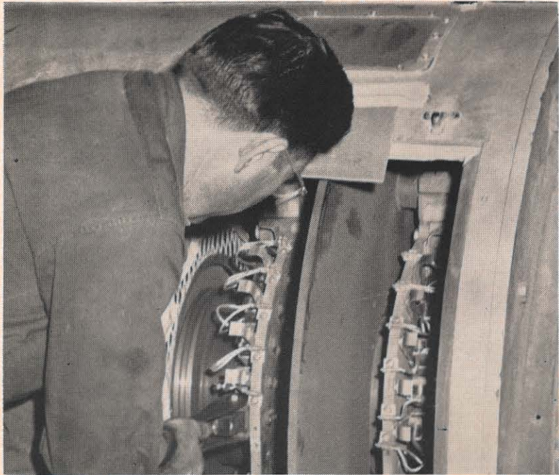
A new tool has been developed at Kanawha River plant that permits maintenance men to true generator collector rings with the unit spinning at full load. Before it had been necessary to slow the generator or stop it completely to do the job. Jack Crist, master maintenance man, demonstrates the tool.
