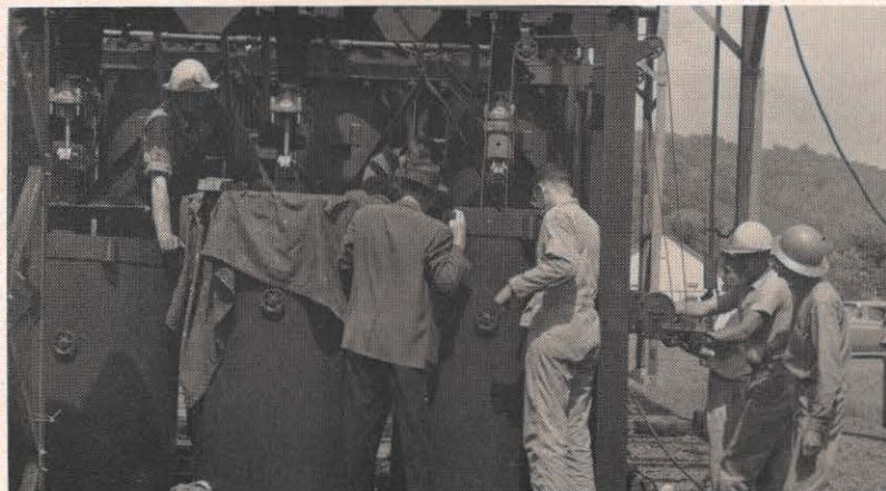
The first step in a program that will see 18 more 69-kv breakers installed in the Pikeville district was completed recently. Two breakers were installed in the Betsy Layne station and checked by factory representatives, system and local station employees.
