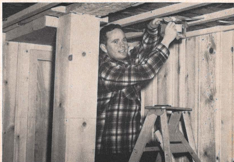
Earl Driskill, handyman. Here he wires a ceiling fixture for his finished basement room, which he did entirely by himself.
