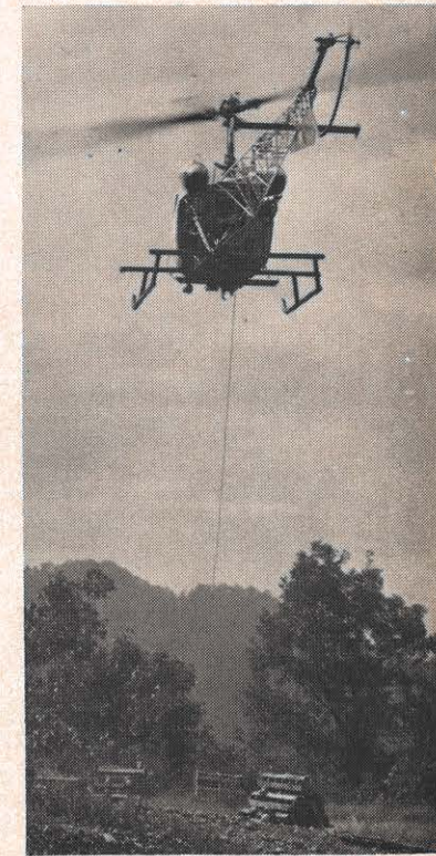
Picking up a bundle of insulators, the helicopter prepares to carry them to a practically inaccessible pole in the Williamson district.
