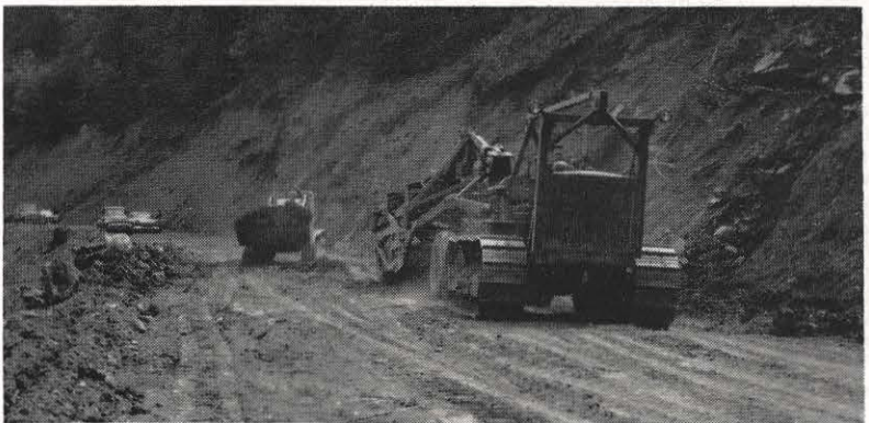
A road is being built in West Virginia to replace one in Virginia. This is the work going on in Glen Lyn, where a road is being cut as part of a new flyash dike, and the state line wanders almost at whim through the area.
