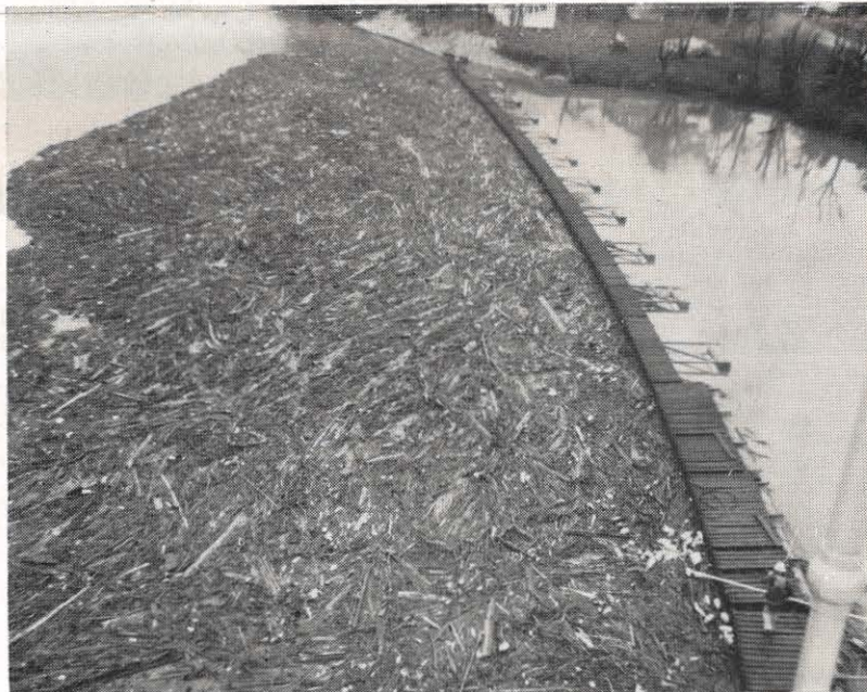
Heavy rains and spring floods brought the usual problems at Kanawha Valley Power Company's hydro installations near Charleston. Log jams such as this first strike London plant, then Marmet about a day and a half later, and two days after that, Winfield, 50 miles downstream. The logs and trash are diverted through the rollers to move it on.
