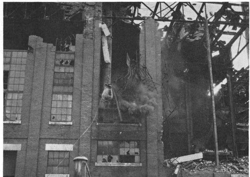
A huge and weighty ball of concrete, swung from a crane, undertakes the work of knocking down the old Kenova steam plant at Kenova in the Huntington division. The plant was retired several years ago, and salvage and demolition work was started recently.
