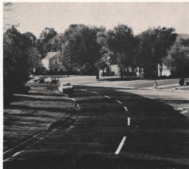
The use of fly ash as both a filler in asphaltic concrete for black top roads, such as this one, and as a sub-base for highway construction was approved by the Bureau of Public Roads as far back as 1952.
