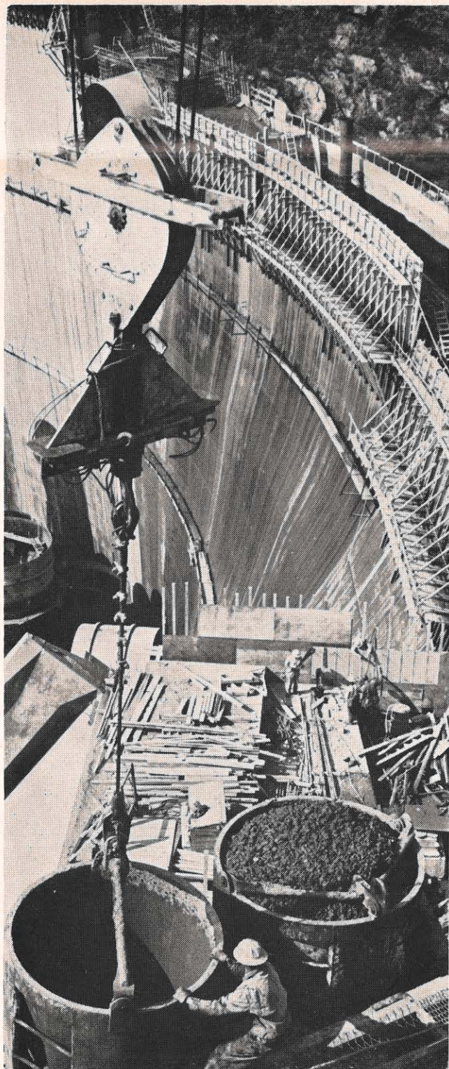
All major construction on the AEP System used fly ash, and great quantities were added to concrete mix at Smith Mountain Dam, above, and to Cardinal plant. At the present time, fly ash is being used in the construction of Muskingum plant Unit 5 and Big Sandy plant Unit 2.
