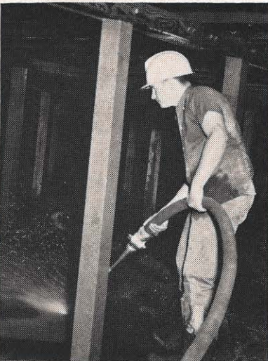
During the recent two-week planned outage of Clinch River's Unit 3, extensive maintenance included replacement of refractory in the ash hopper, and above, cleaning mud accumulation from the base of the cooling tower.
