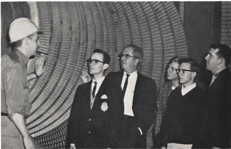
C. T. Brooks, assistant results engineer at Kanawha River plant, explains the components of an intermediate pressure turbine rotor to John E. Miles, assistant director of engineering at West Virginia Institute of Technology, and four senior mechanical engineering students. Forty engineering students took advantage of a recent outage at the plant to observe major equipment undergoing repair. The students inspected internal parts of a turbine-generator unit and observed a major re-tubing job in a boiler. They received classroom credit for the tours.
