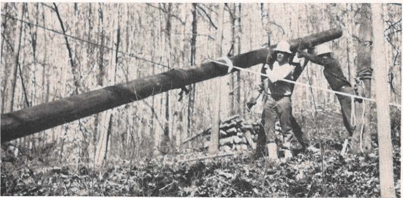
Crew members begin raising the pole with the help of the winch line. The tree behind the men was the anchor point for the winch line.
