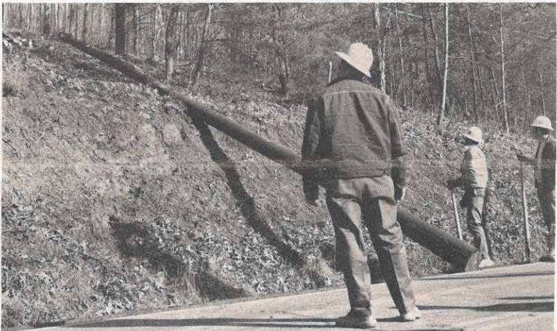
The pole begins its way up the hillside, thanks to a unique pulley and winch system.
