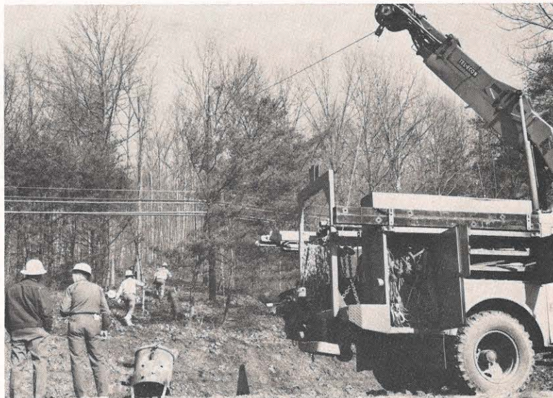
John Moss and Bus Shaffer, line foremen, converse as the pole moves ahead. Note the winch line from the truck boom traveling across the road to a pulley mounted on an existing pole.
