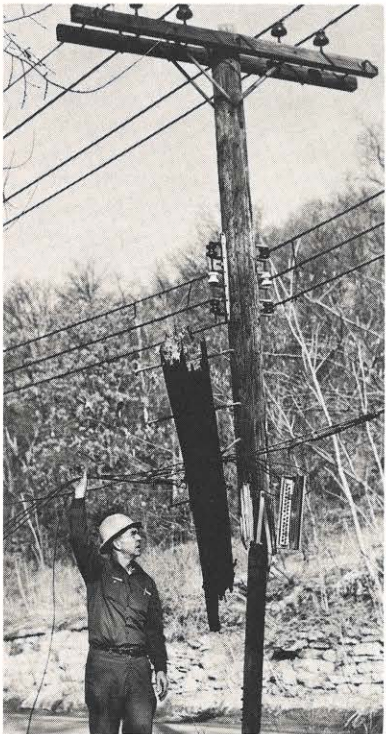
HANG IN THERE—C. C. Harper, Charleston meter serviceman A, holds broken wires as he tries to figure out how primary electric service was maintained after a car struck this pole.
