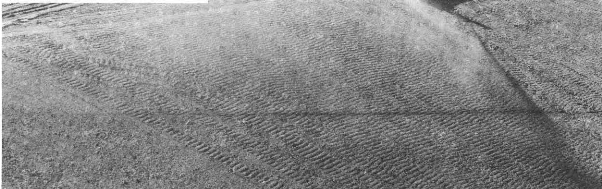
A close-up view of the hydro-seeding of a mountain top after its terrain has been gently rolled. Grass seed, together with fertilizer, is mixed with water and "blown" by pressure nozzles to cover large areas. Within days the greenery is restored.
