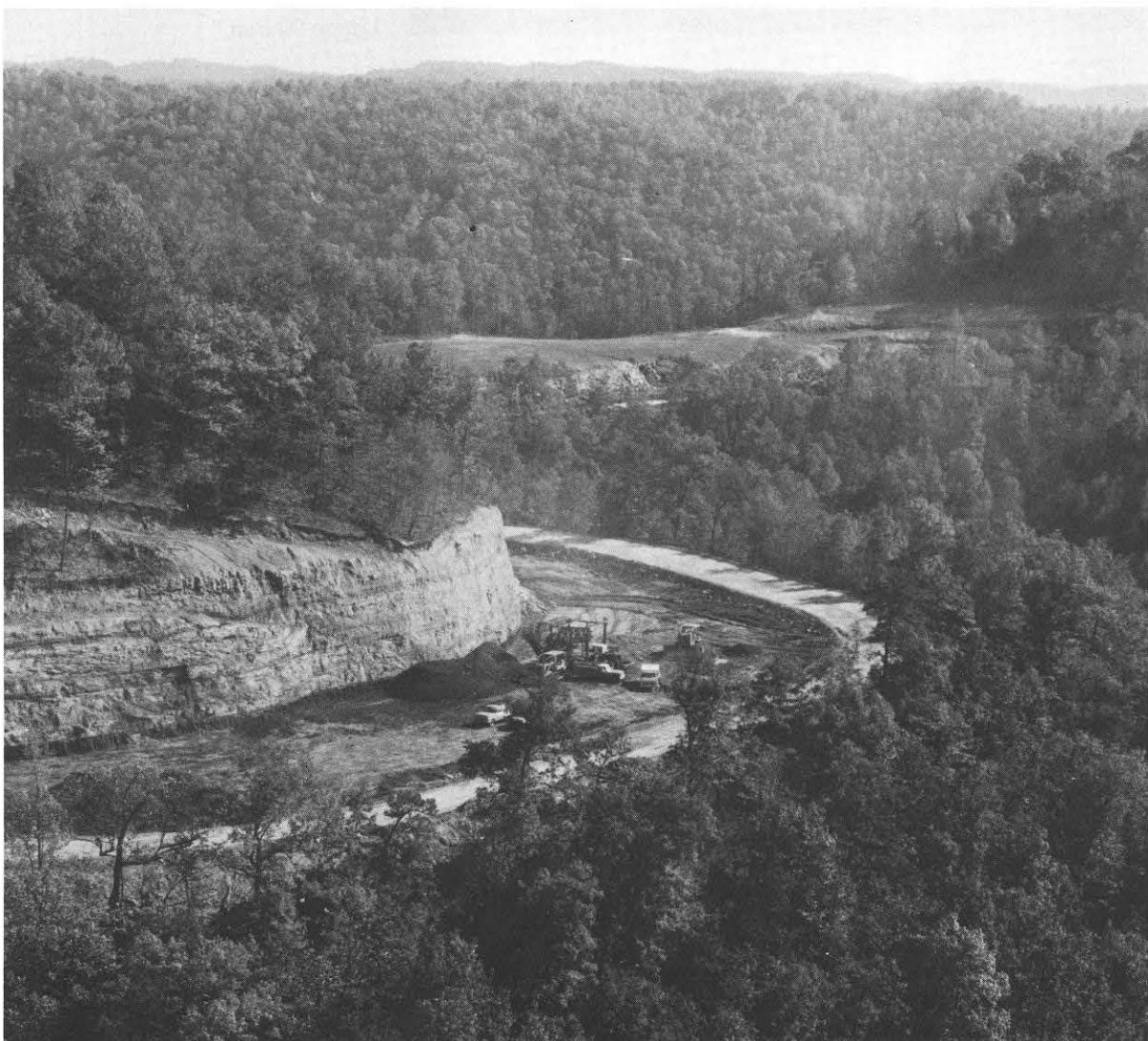
Here is an over-all view showing the "terrace" cut and mining in the foreground and the reclamation results from previous mining in the background.
