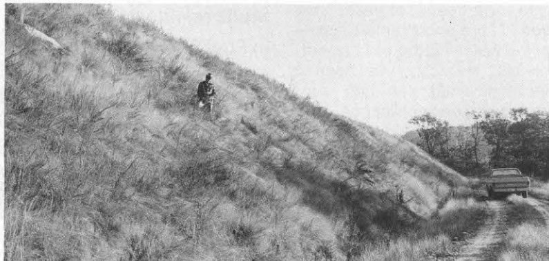
After the coal is removed, the stored topsoil is returned, a gentle slope is created and grass is planted. This photo was taken only months after the mining.
