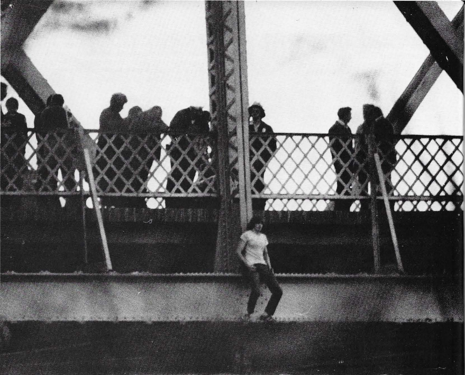
A troubled young man stands precariously on the ledge of the 6th Street Bridge as firefighters try in vain to talk him out of jumping into the Ohio River.
