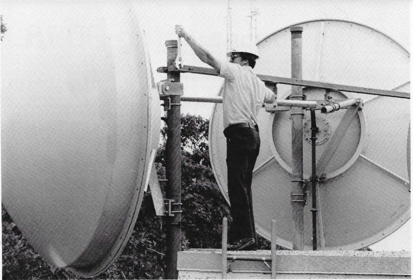
Lou Sturm, engineering technologist, GO T&D Communications, Roanoke, on the roof of the Poor Mountain MW-1 microwave site, makes an adjustment to the antenna path alignment.
