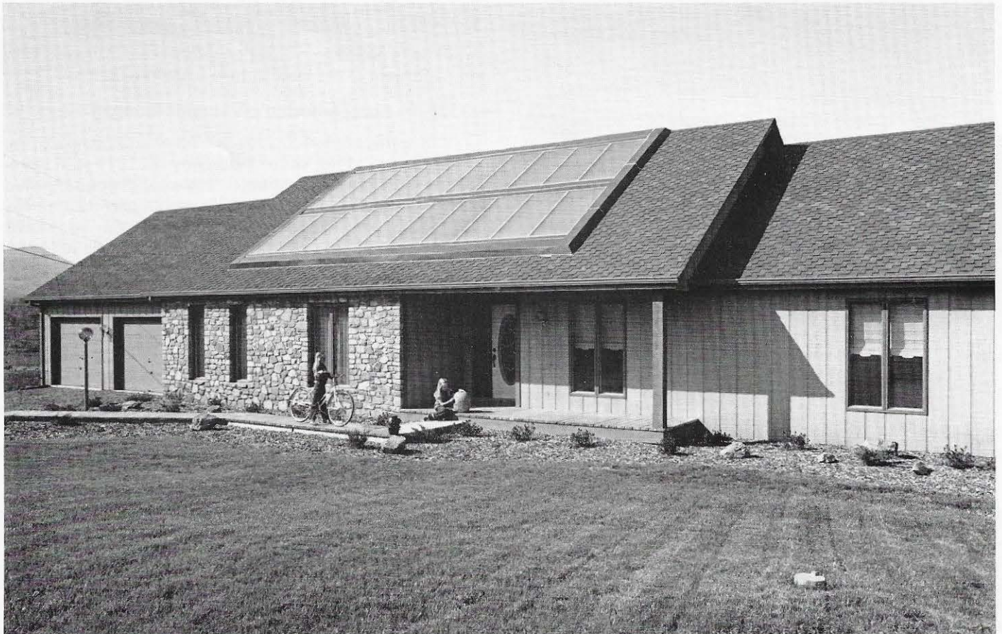
This is one of two solar heat pump test homes constructed as part of Appalachian Power Company's residential energy conservation program. Located in Botetourt County, near Roanoke, Virginia, it is the only house in the American Electric Power service area where a solar heat pump, domestic hot water system and off-peak energy storage are combined. Appalachian's other test home is located in Hurricane, West Virginia.
