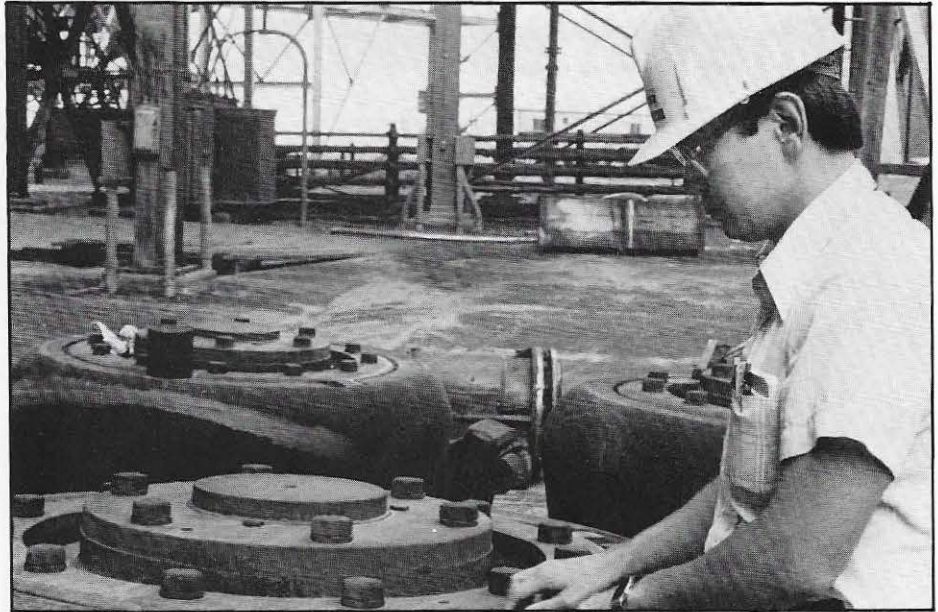
Amos Unit 1 Outage Coordinator Duane Phlegar examines rollers from one of the unit's six pulverizers. In each pulverizer, three rollers crush incoming coal to a fine dust before combustion. All of the pulverizers were reconditioned during the outage this year.
