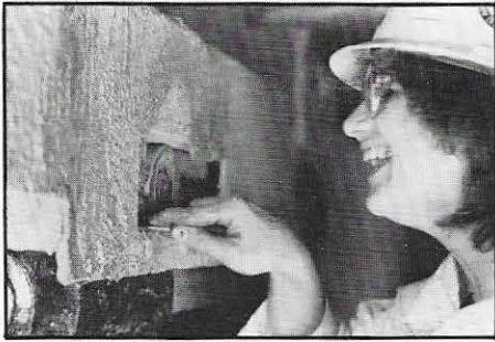
Utility Worker Beth Smith tackles buildup on the Unit 1 slag blowers during the maintenance outage.
