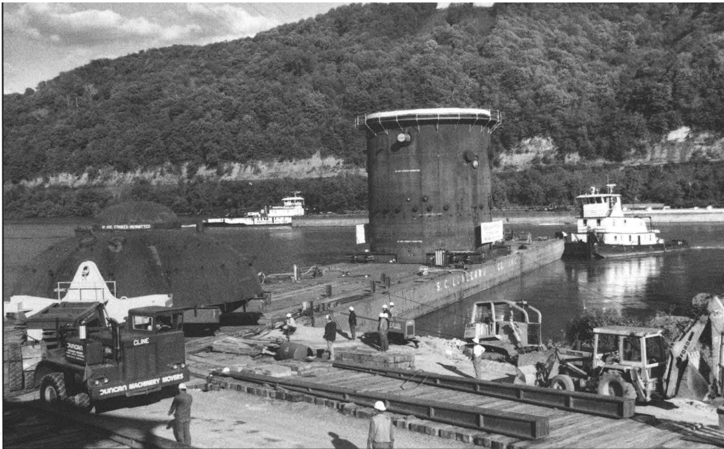
The combustor vessel, with its 17-foot high hemispherical head detached for clearance under bridges along the route, is loaded onto a 276-foot oceangoing barge owned by the S. C. Loveland Co. Inc.
