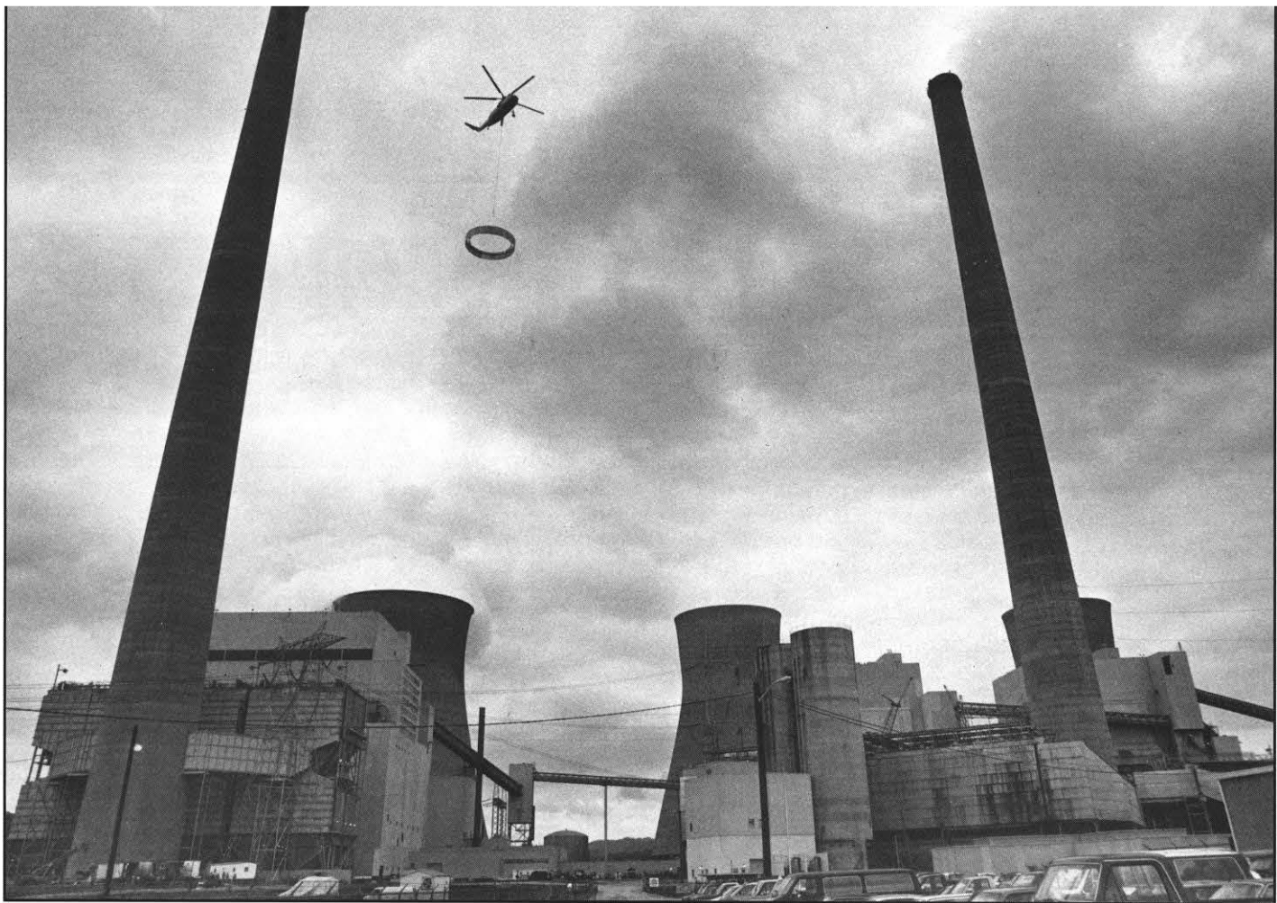
The helicopter, which was used to replace the stainless steel liner for the stack serving Units 1 and 2, hovers over the John E. Amos Plant. Photo courtesy Chet Hawes, Charleston Daily Mail.
