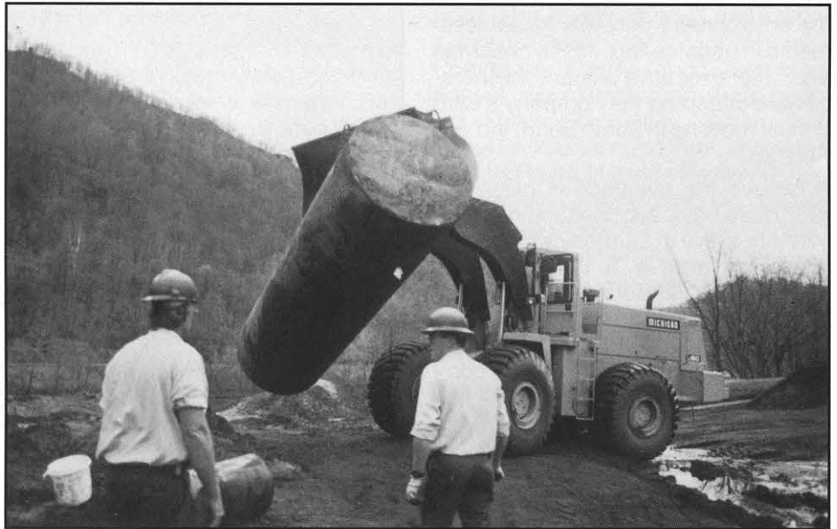
Existing UST at Kanawha River Plant's coal yard is removed from excavation.
