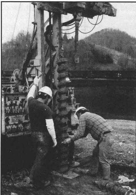
Hydrogeological contractors begin installation of groundwater monitoring wells at Clinch River Plant's UST project site.
