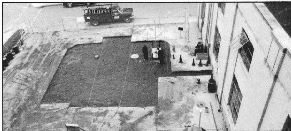
With engineered backfill compacted and in place, contractors set dispenser island and prepare for concrete pavement construction at the Virginia Street office.
