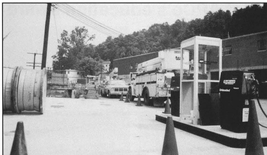
Newly installed UST facility at the Fieldale office awaits completion of concrete curing.
