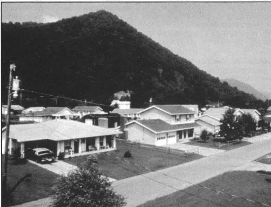
Nearly 100 homes were built on a fly ash structural fill at the Adena site in West Virginia.
