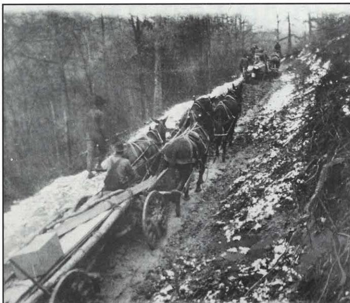
**In the 1920s, oxen carried steel used in the construction of transmission towers up the mountainsides.**
