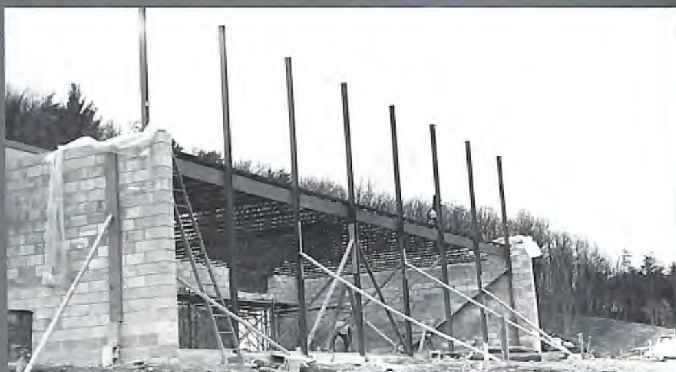
1973: Addition to Upper School under construction
