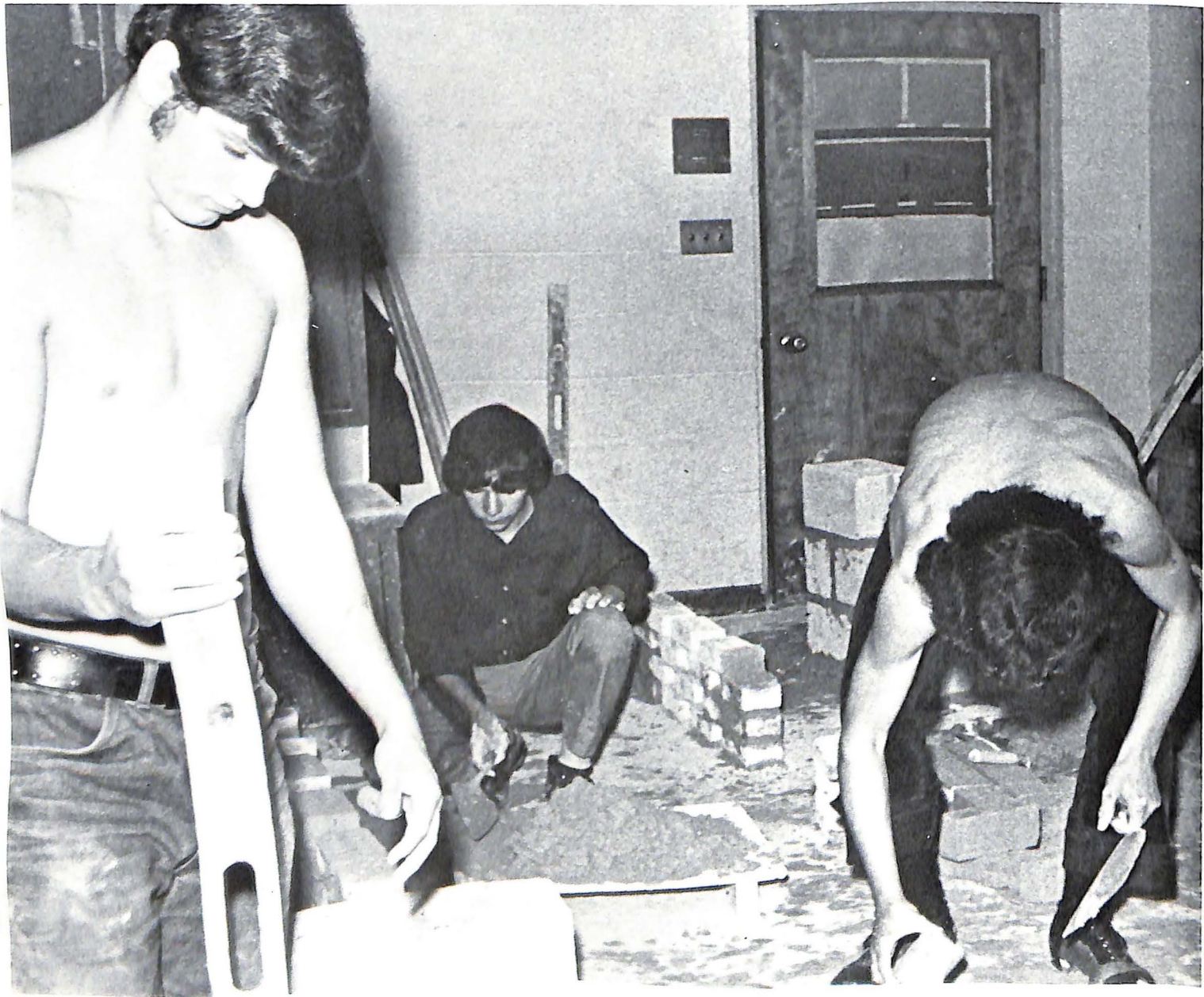
MASONRY STUDENTS Sam Robinson, Jim Conner, and Mike Scott learn the art of bricklaying by building fake walls, using a mixture of clay and sand instead of cement.
