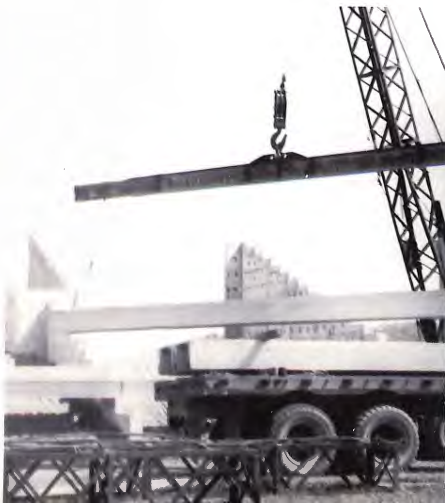
Northside's stadium goes up.
