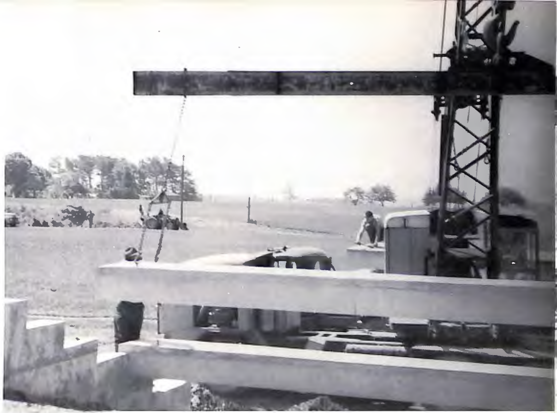
Crane lifts seats into place for our new stadium.
